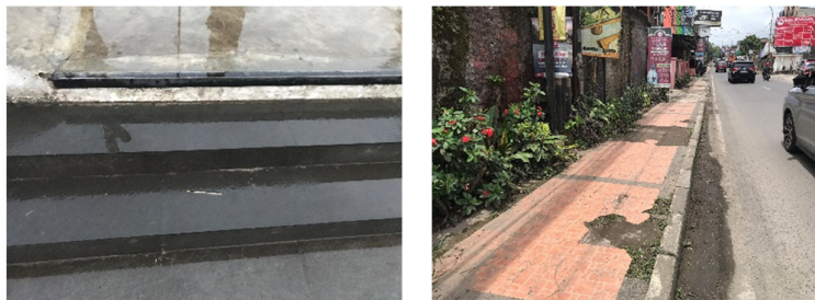
Figure 4. Pedestrian Way Surface along Lembang Street Segment
