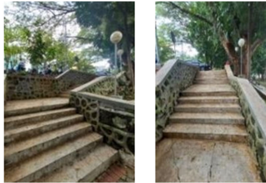
Figure 8. Concrete Railing Source: Author, 2025
