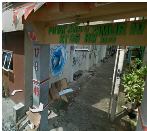
Gambar 4 Kondisi Drainase Sumber : Google Earth, 2021
