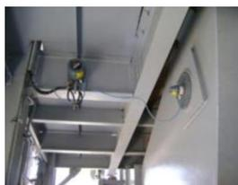
Gambar.3. *Chute Block Switch*
