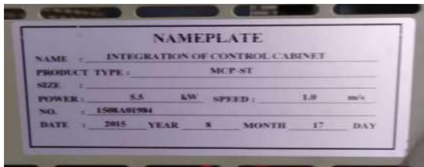
**Gambar 5.** Name plate sistem kontrol lift
