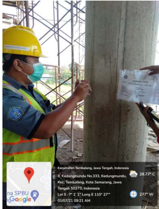
Fig. 8. Implementation of the Hammer Test
