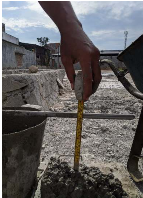
Fig. 9. Slump testing in the casting
