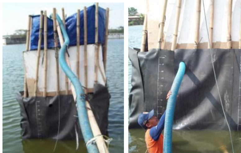
Figure 4. All instrument was installed to the pontoon and sinking process of pontoon [10]
