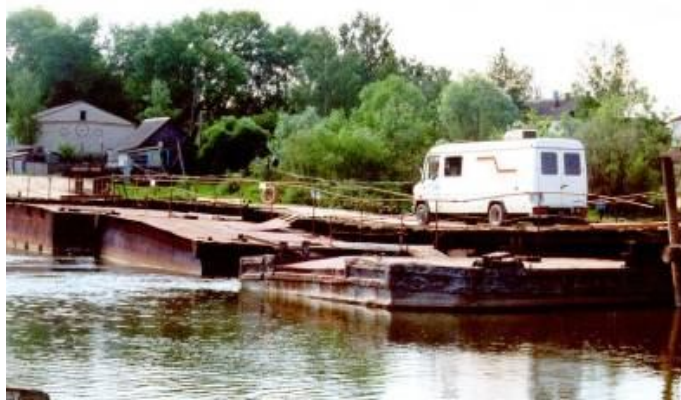
Fig. 1. Pontoon foundation with bridge decks
