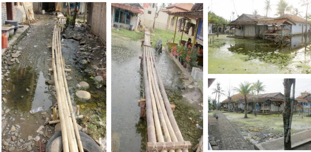
Figure 3. Streets Construction Source: Observation and in Depth Interview, 2015
