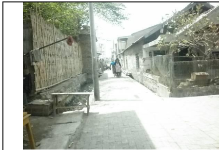
Figure 8. Paving road conditions
