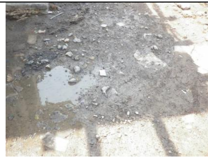
Figure 9. Dirt road conditins
