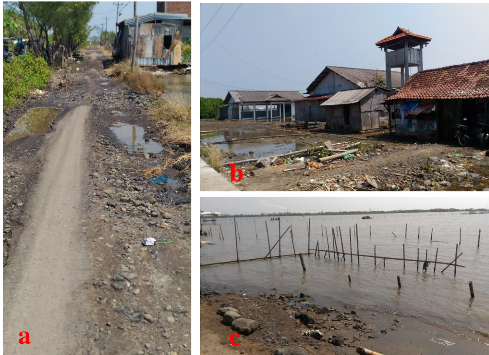
Fig 3. Facilities damage in Kelurahan Mangunharjo caused by tidal and abrasion
