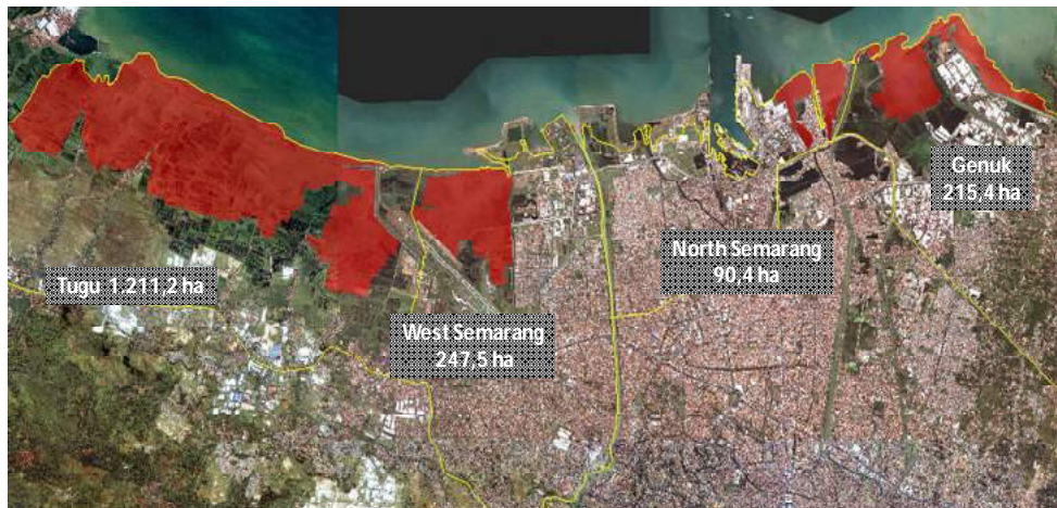
Figure 9. Erosion of Semarang Coastal Area (Anggoro, et al, 2014)
